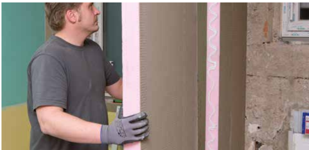
2. Now it is immediately possible to join one Murexin Uniplatte to the next.
