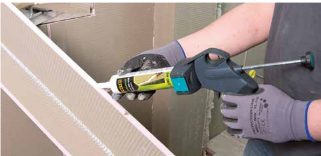
1. Paint the edges of the board with Special Adhesive X-Bond MS-K88 Express .
