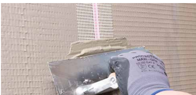
4. Insert the Glass Fibre Fabric GS 10 , simply fill with Murexin adhesive mortar – the substrate is ready!
