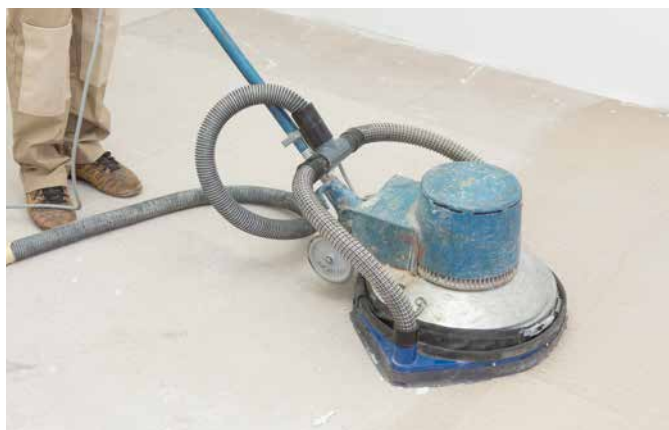
Substrate milled, shot blasted or ground according to ÖNORM B 2236, DIN 18356.
