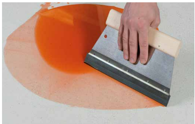
Barrier created with MUREXIN Silane Moisture Barrier MS-X 3 or Silane Bonding Resin MS-X 1
